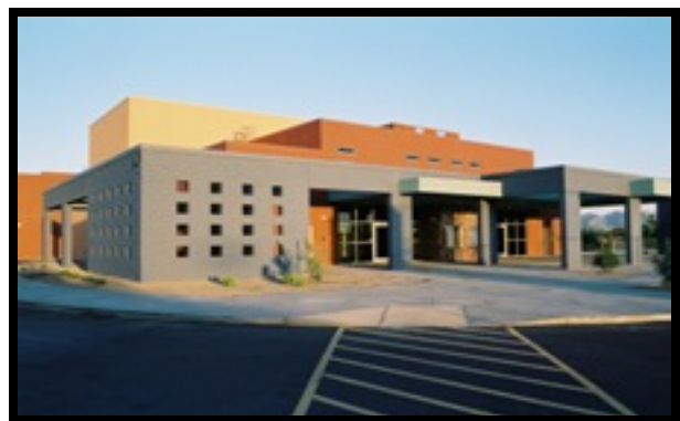
Desert Edge High School Valley high school is fifth in the world to earn LEED Silver certification!
